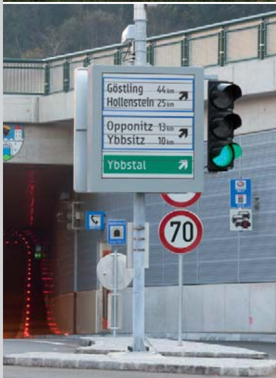
Buchenberg Tunnel, Waidhofen/Ybbs, Austria
